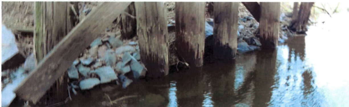
Bent 3 decayed piles
