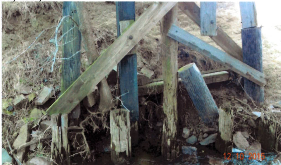
Timber Piling-failing and severely decayed
