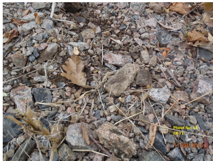
Typical ballast found on existing rail corridor.
