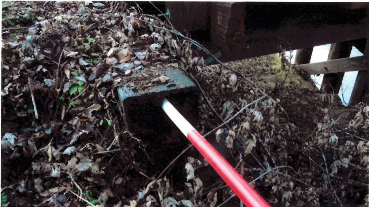
Decayed Abutment Backwall Plank
