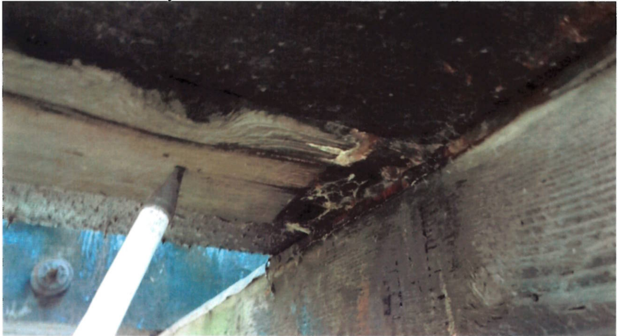
Timber Stringers-Decay at the ends
